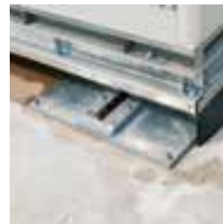
Seismic isolator for shelters
