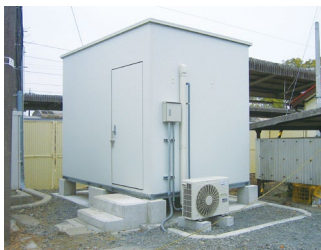
Shelter for signals/communications
