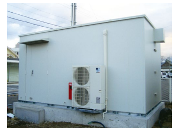
Shelter for disaster prevention wireless system
